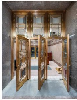
Brass doors in the historic Senate Office Building are included in a broader effort to conserve the building's historic entrances.
