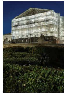
The west facade of the Supreme Court of the United States illuminated at night, with scaffolding in place for exterior restoration work.
